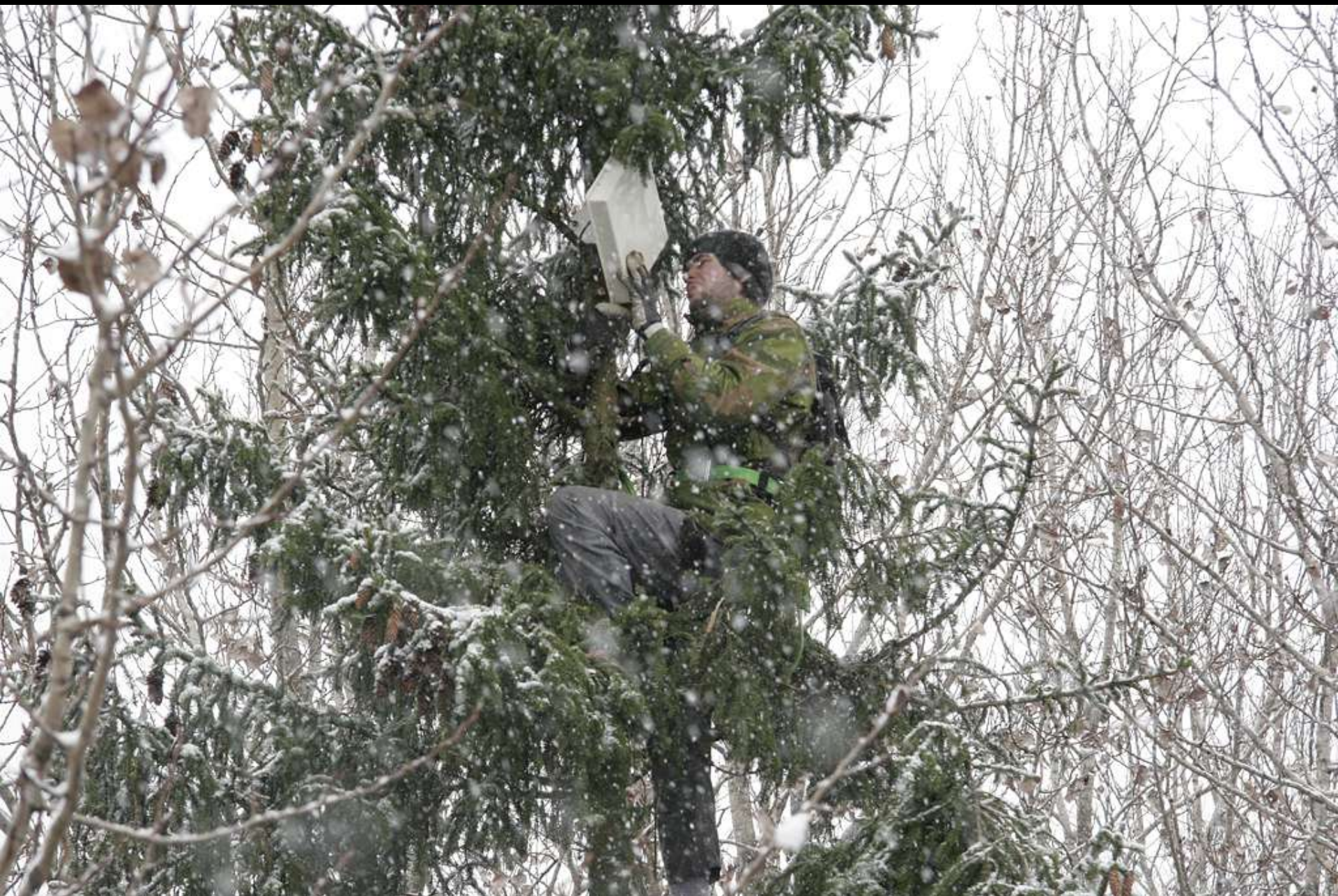
Install of antennas, good weather because eagles do not see us
